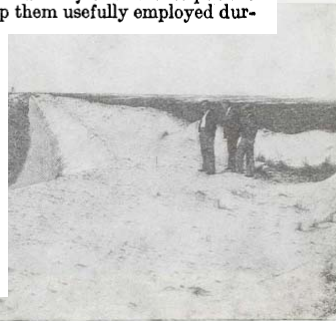
FIGURE 48.—Main drainage ditch through sandy soil, Cat Island, Miss., dug by C. W. A. workers as a mosquito-control measure.
