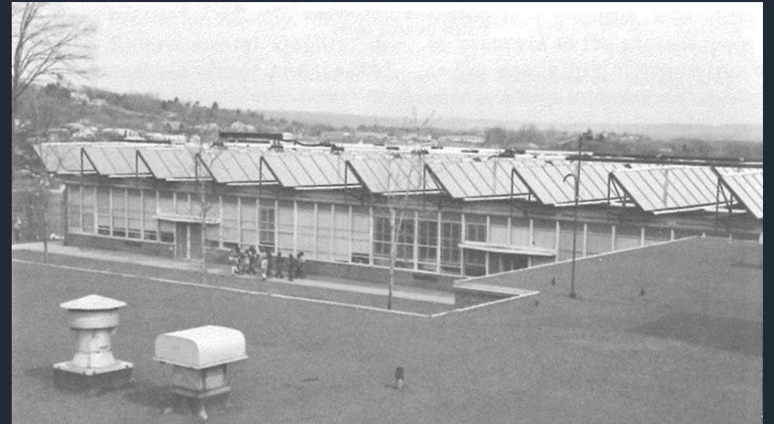
Timonium elementary School near Baltimore became the first school in the U.S. to be heated by solar energy in 1974 as part of NSF's solar energy program of RANN.
