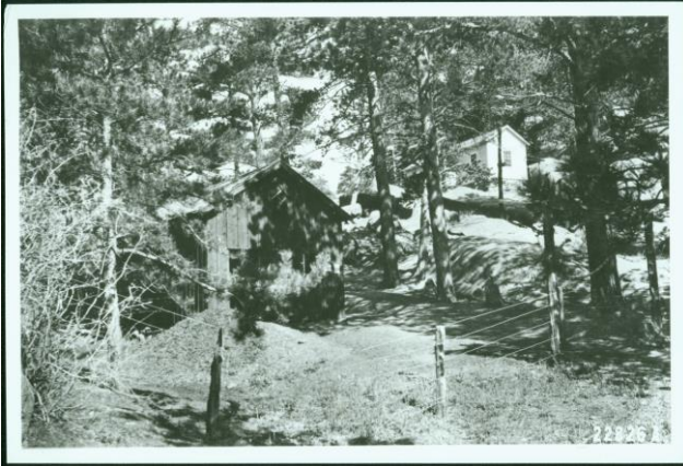
Outbuildings of Old Man Mountain Ranger Station Circa 1915.
