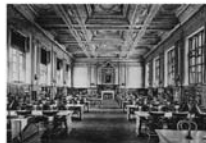
View of the interior of the Depository Building in St. Louis, Missouri, designed by Hugh Wilson.
