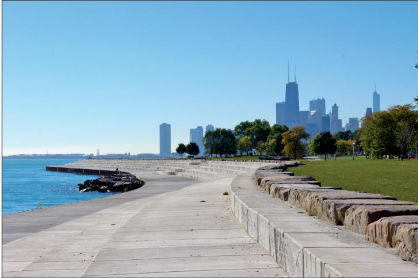
Restoring Chicago's shoreline protection (Chicago District)
