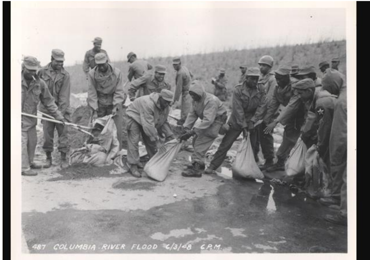
National Archives photo of soldiers filling sandbags during Vanport Flood-Columbia River, near Portland, OR (June 3, 1948)
